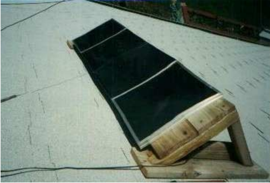
Solar panel on the roof
