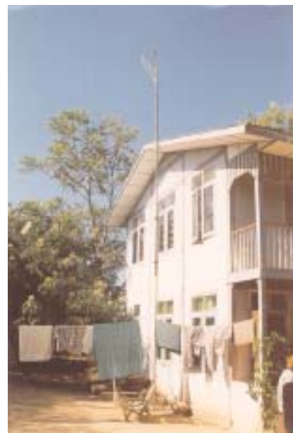
interWAVE's Deployment of a Yagi Antenna
