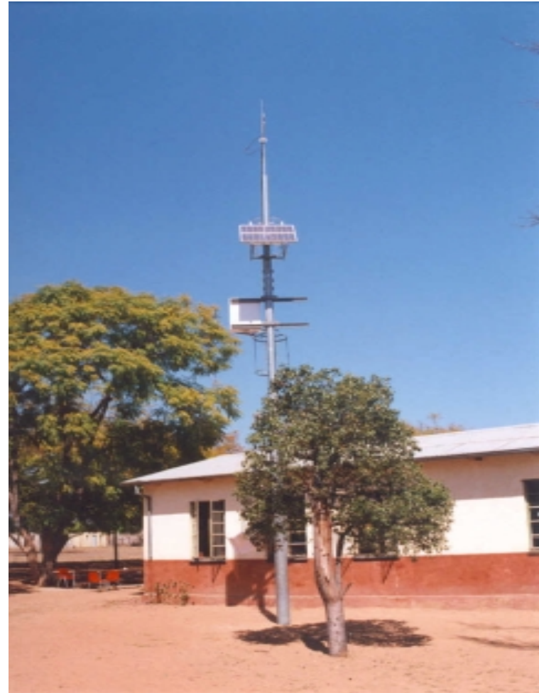
Telkom VSAT installation for 1994 elections. Matopas, Northern Province South Africa
