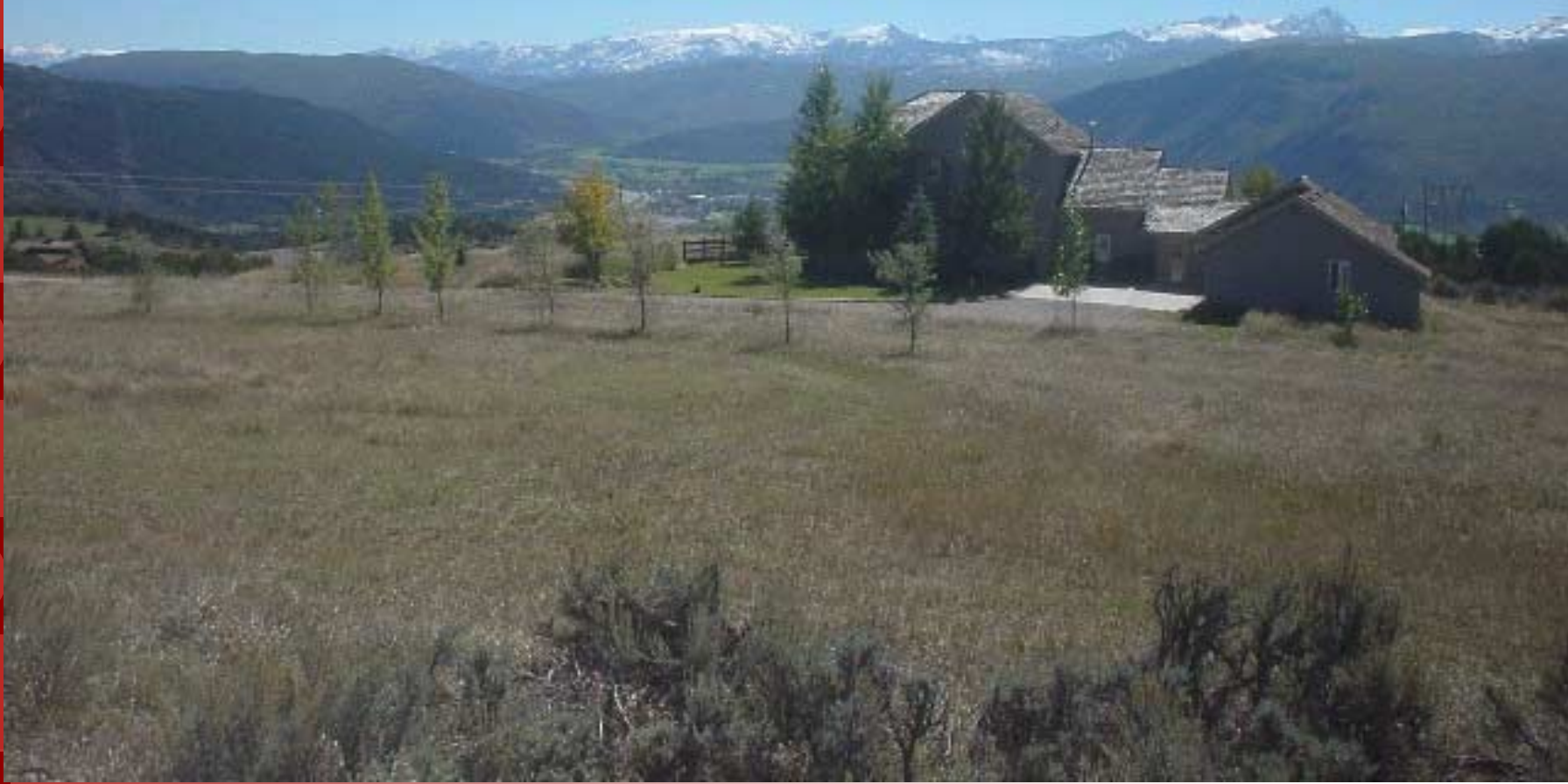
House with repeater near Aspen Colorado
